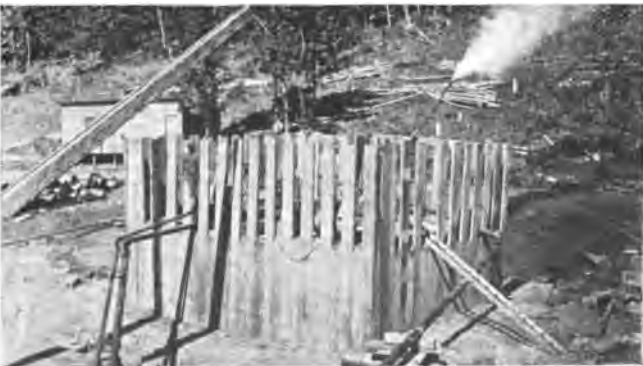
C. SINKING SHAFT IN OVERBURDEN, SOUTH LAKE MINE, 1911.
